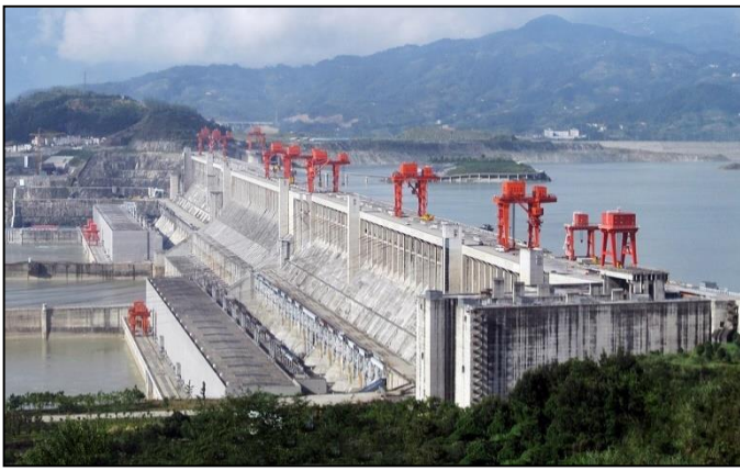
Three Gorges Dam on the Yangtze river is the largest hydroelectric power station in the world
